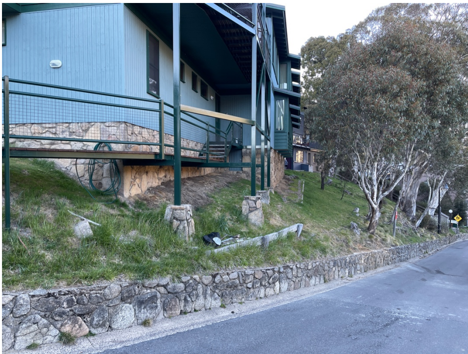
Photo 2 View of existing ramp and walkway
